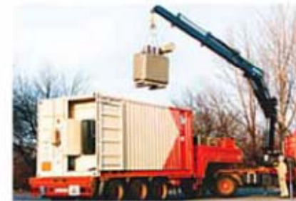
Utovar transformatora
